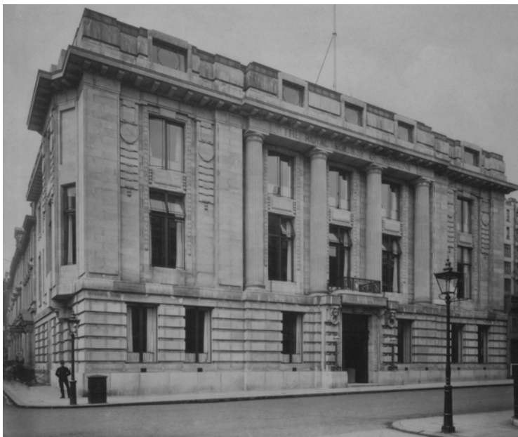
Royal Society of Medicine building, site of the 4th ILAE meeting in August 1913. The building was opened in May 1912 by King George V and Queen Mary. The society was formed in 1805, with the aim of promoting ‘conversation on professional subjects, for the reception of communications and for the formation of a library’. The library housed in this building is now one of the best medical libraries in the world. (By kind permission of The Royal Society of Medicine)
